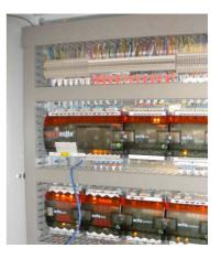
The new BMS system installed has proven to be reliable dispensing with numerous call outs the site generated previously, energy efficiency is also noticeable with the building manager now trimming on/off times to suit the building, weather etc which was not possible with the old system.
