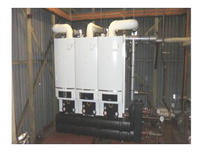
CBAC Services Ltd installed 3 new Buderus boilers on a cascade system in the roof top plant room. This was due to the existing boilers failing during the winter months, as diagnosed the heat exchangers where severely damaged due to frost protection failing, parts were no longer available.
