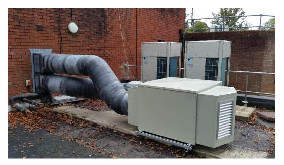
CBAC Services Ltd installed a new Daikin VAM fresh / extract unit and VRV to the 1st floor Force Control room.
