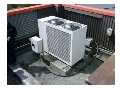
CBAC Services Ltd installed a new AERMEC 47kw air cooled chiller as a replacement for the existing Trane unit which had failed due to the age of the unit and had been unreliable for many years resulting in costly repair works.
