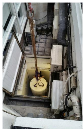
This particular tank is made from stainless steel, insulated and can take mains water pressure to the max of 6bar. The max kilowatt of heating it can have is 57 so the manufacture recommended us fitting 1 x 12kw in the upper port and 1 x 45kw in the lower port.
